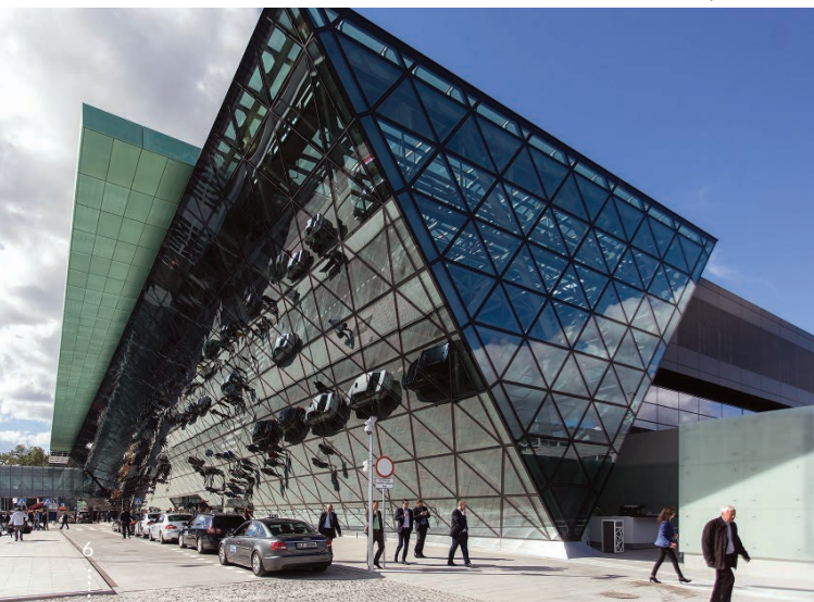
Kraków-Balice International Airport
